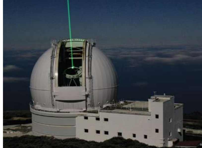
◀ A Rayleigh laser guide star is launched from the William Herschel Telescope on La Palma to probe the atmospheric conditions above the telescope for adaptive optics.
